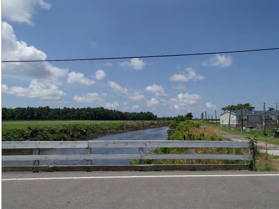
Figure 22: East Main Canal, facing southwest across Bridge No. 21
