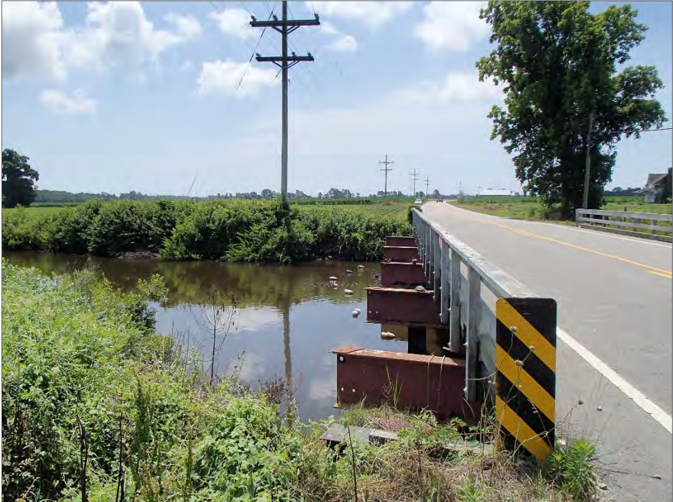
Figure 21: East Main Canal and northeast side of Bridge No. 21
