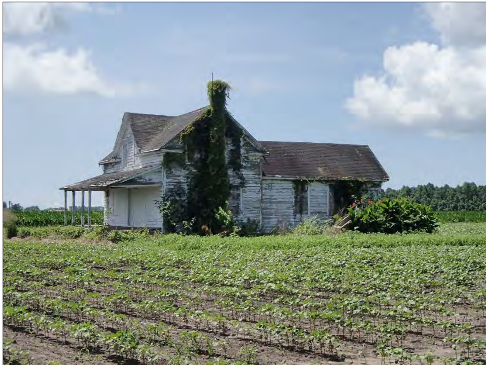
Figure 13: Cahoon House, northwest elevation
