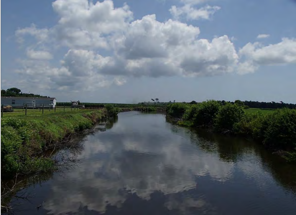
Figure 20: East Main Canal, facing northeast from Bridge No. 21
