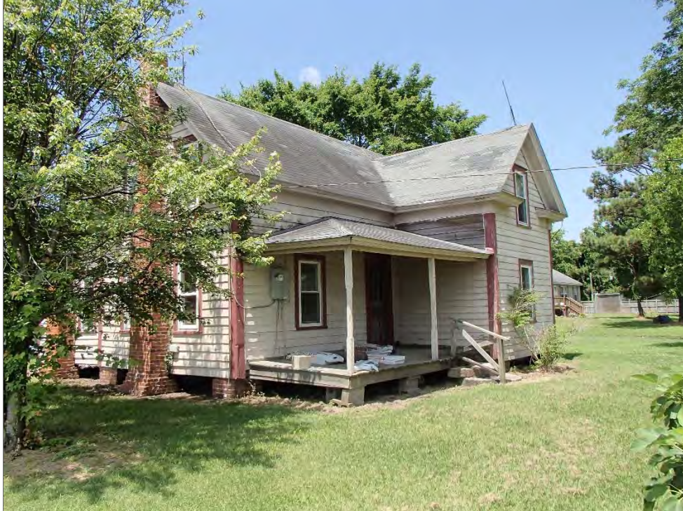
Figure 7: Davis-Gibbs House, east corner
