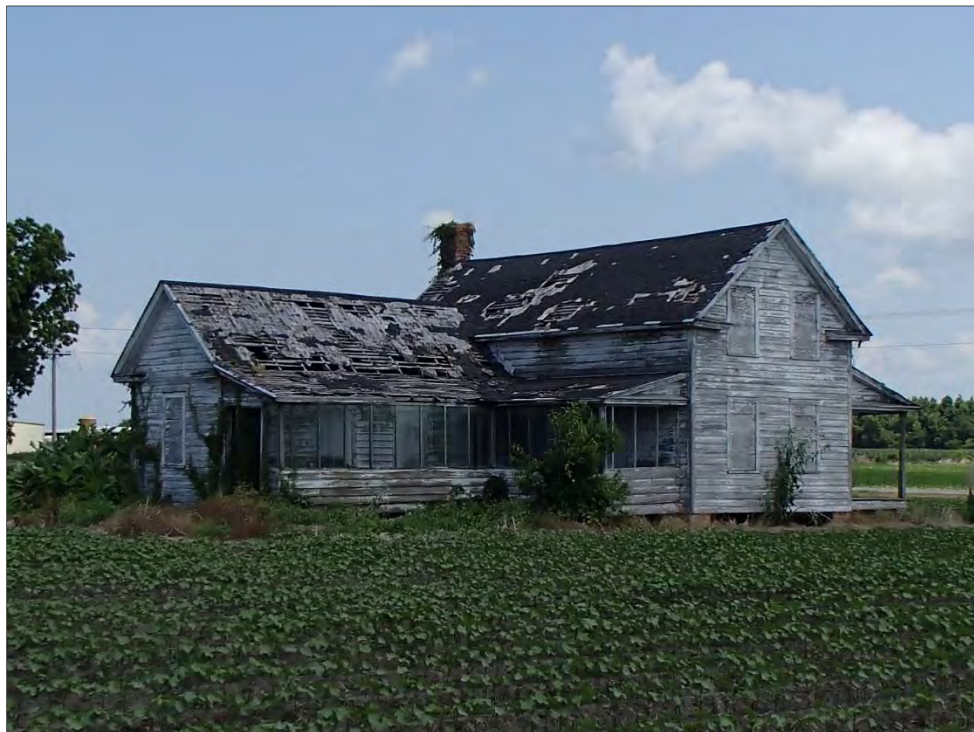
Figure 15: Cahoon House, south elevation
