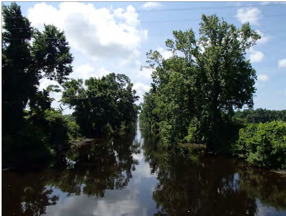
Figure 25: Outfall Canal, facing south from U.S. Highway 264
