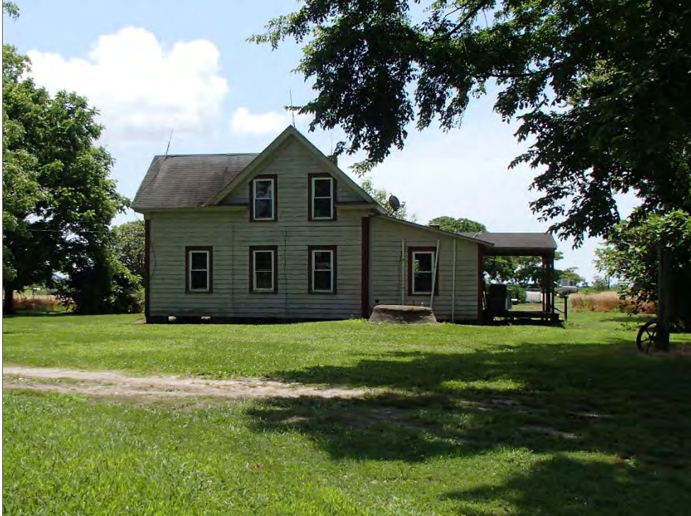
Figure 5: Davis-Gibbs House, northwest elevation
