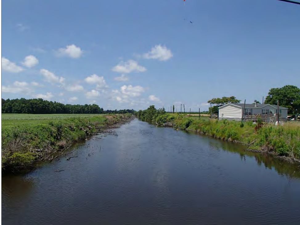
Figure 18: East Main Canal, facing southwest from Bridge No. 21
