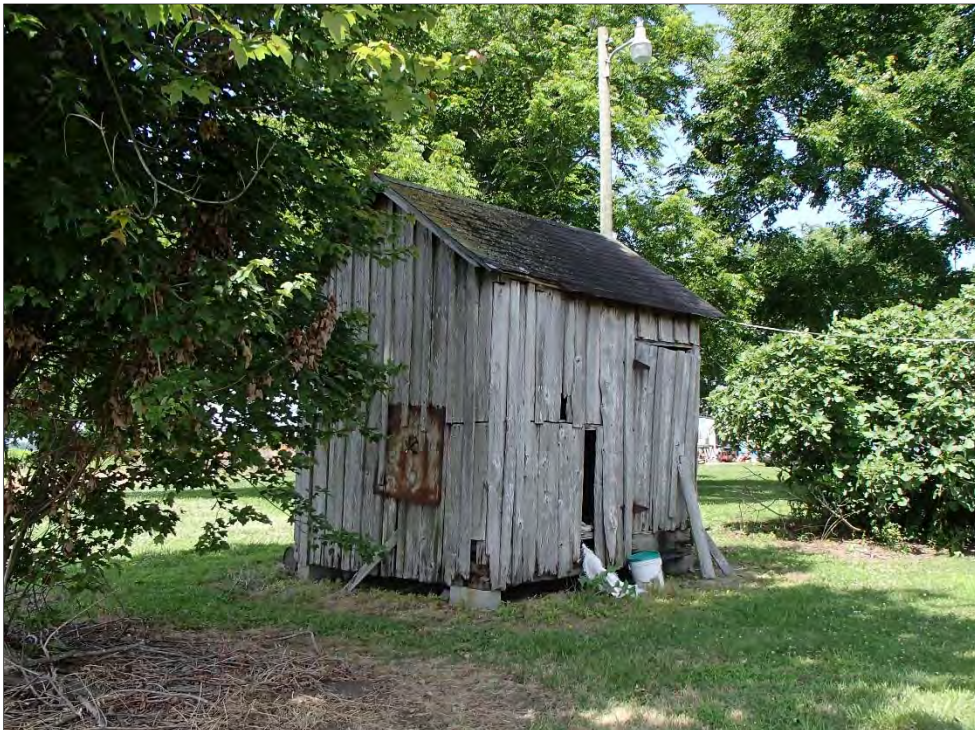
Figure 8: Davis-Gibbs House, former kitchen/barn, east corner
