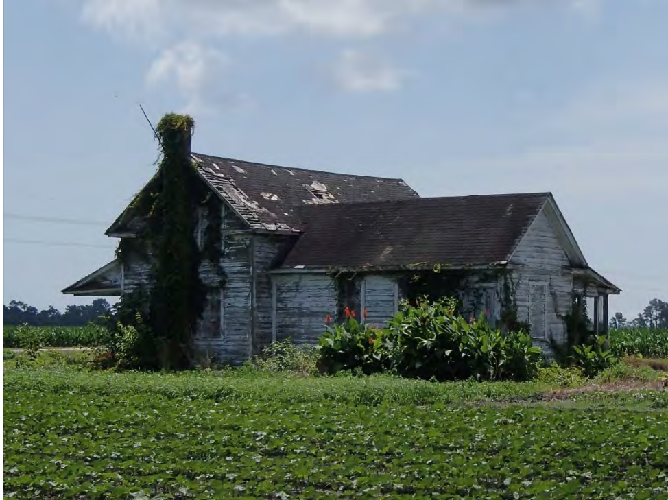
Figure 14: Cahoon House, northwest elevation
