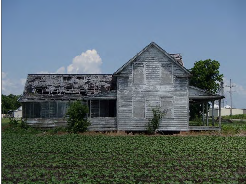
Figure 16: Cahoon House, southeast elevation
