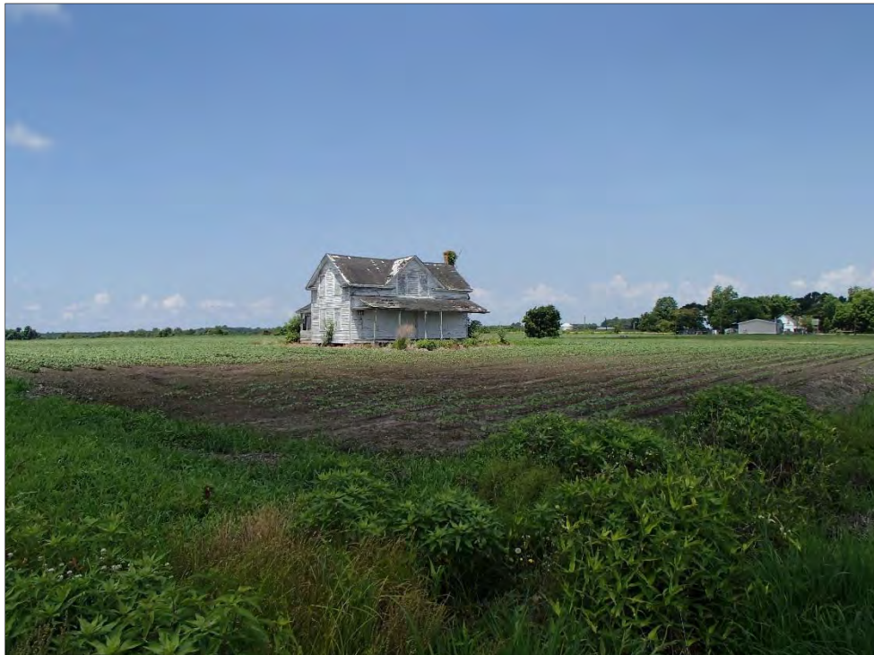
Figure 17: Cahoon House, east corner
